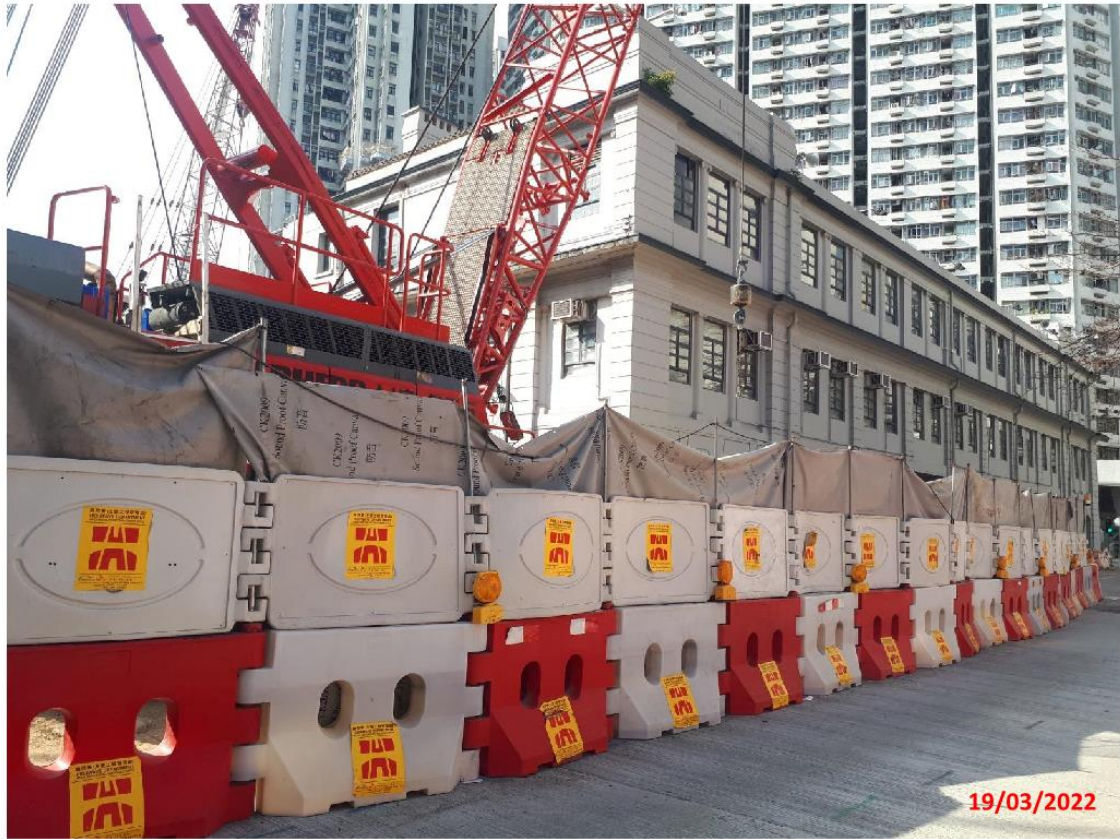
Figure A1 Noise barrier mat erected along site boundary
